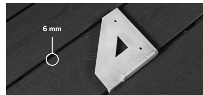
Width-to-Width The required width-to-width gapping is 6 mm.
